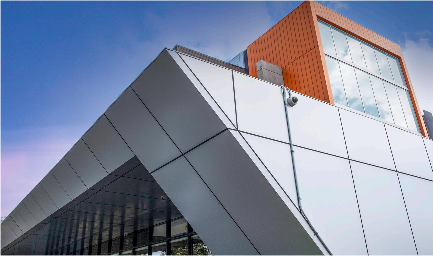
MondoClad® solid aluminium panels have a superior PVDF architectural paint finish that ensures UV stability and colour retention, so that architectural designs will stand the test of time.
