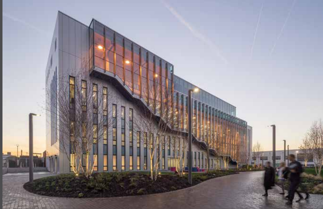
BskyB Believe in Better Centre, UK | Architect: ARUP Associates | Material: ALUCOBOND® PLUS Sunrise Silver Metallic | © Simon Kennedy
