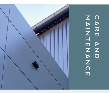
To maintain the high-quality appearance of Nucleo® panels we strongly recommend regular cleaning with a mild detergent and ensuring that any cleaning agents are thoroughly rinsed off the façade.
