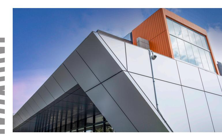
MondoClad® solid aluminium panels have a superior PVDF architectural paint finish that ensures UV stability and colour retention, so that architectural designs will stand the test of time.
